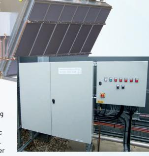
**2: Retrofitting on existing equipment:** Often, as years pass, additional heat load is put into systems, be it industrial manufacturing process or air conditioning applications, meaning existing cooling equipment is no longer able to cope. Adding an adiabatic retrofit package to the existing cooling equipment can solve this problem and avoids the need to spend large sums of money on the strip out of old equipment and the purchase and installation of new equipment.
